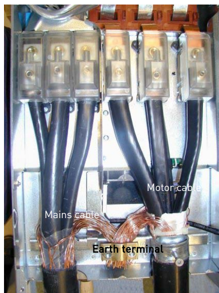
Figure 6-18. Cable installation in Vacon NXS/P, FR8
