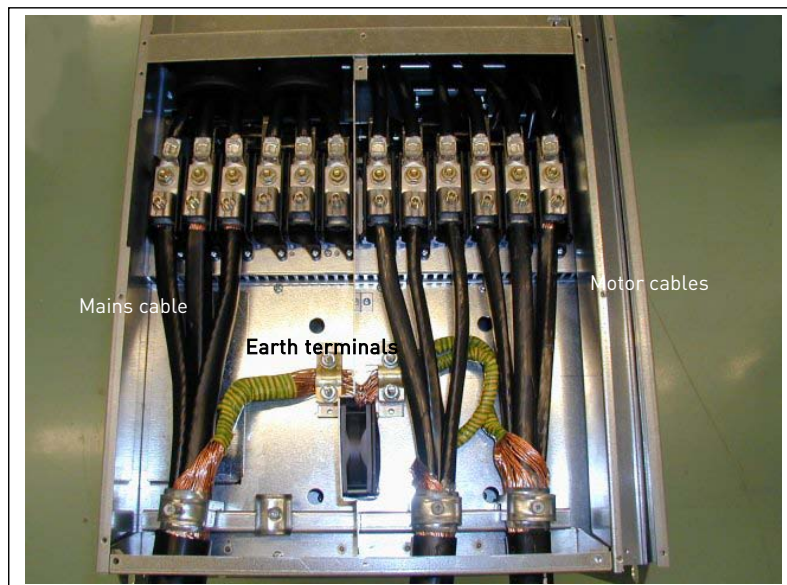
Figure 6-22. Cable installation in Vacon NXS/P, FR9
